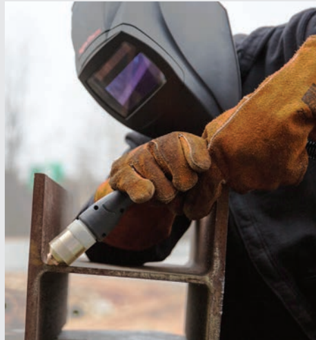
Cut flush to base metal
